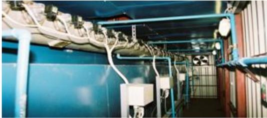
Not only is the pressure low , also the volume is small . But - volume is needed to dislodge the cake from the bag surface. Instead of expensive compressed air we use something which is free : process gas from the clean gas chamber. By right placement of the venturi we get
